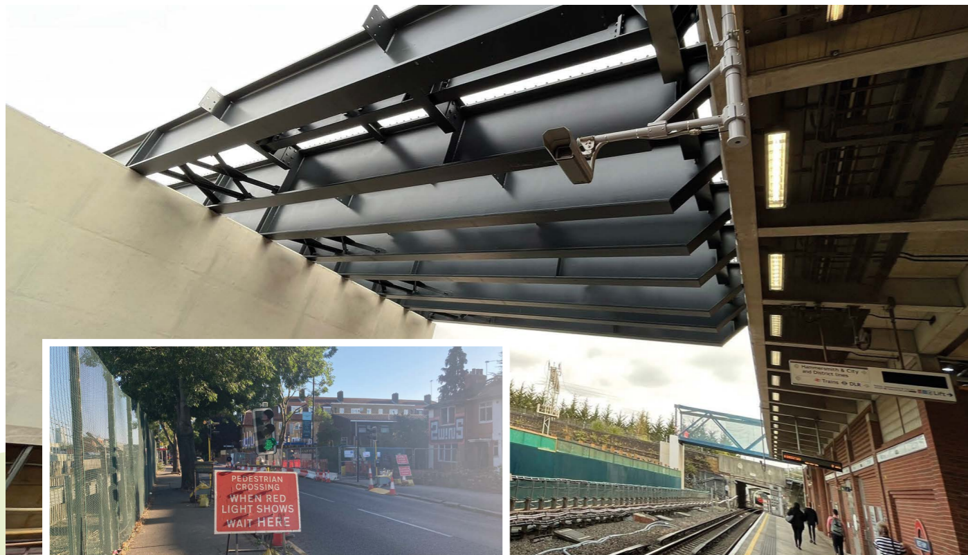
Image of the newly installed station entrance bridge
