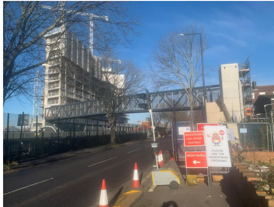
Southern Pedestrian Bridge temporary footpath closure and crossing
